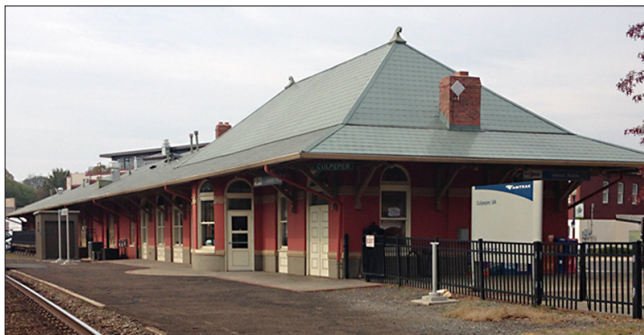
The restored Culpeper depot.
