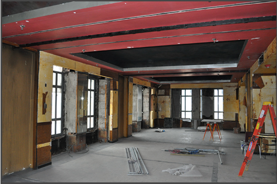
Figure 4. Historic Dining Room – before (Courtesy of CMC)
